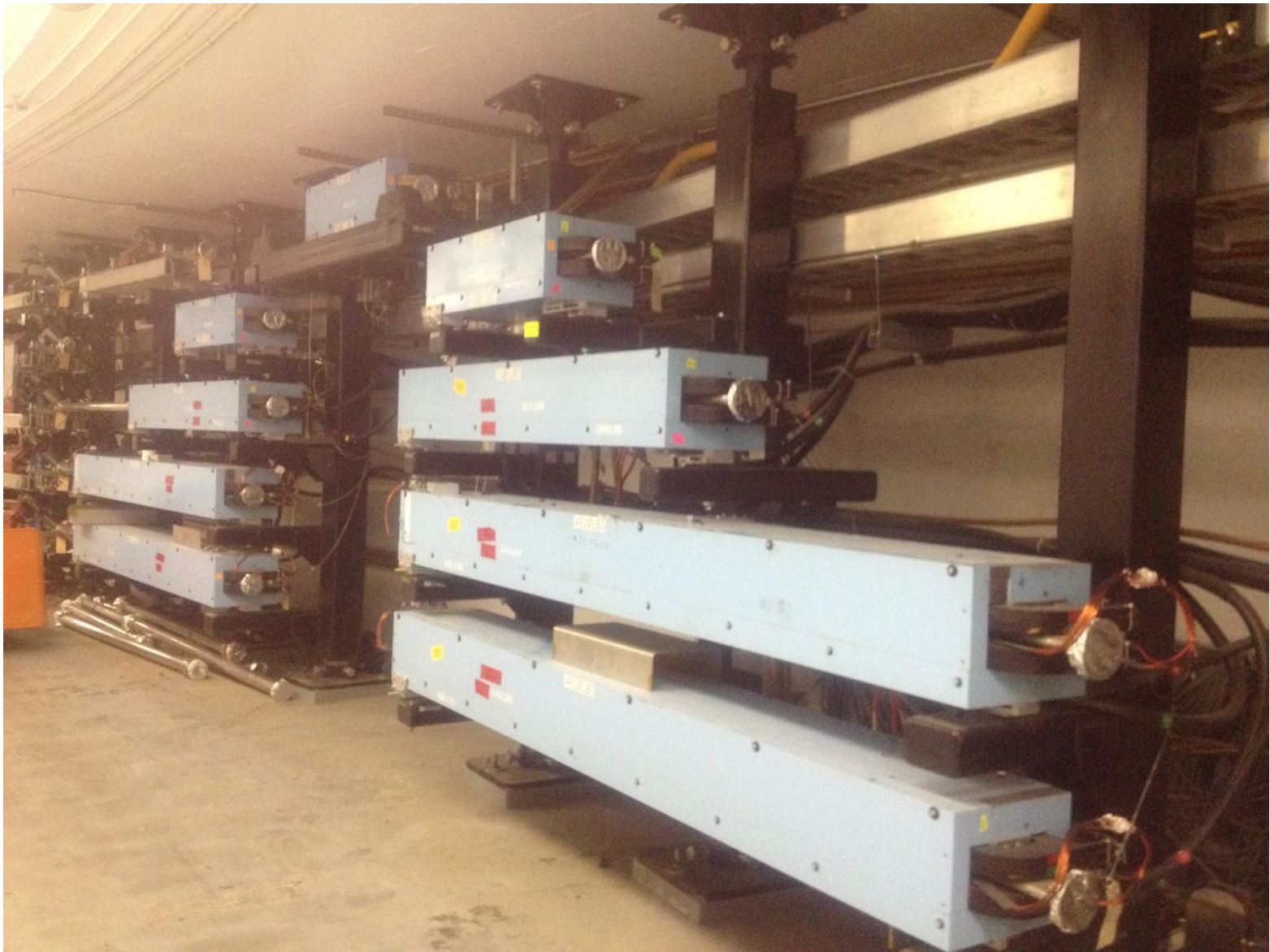
Last Dipole Stack Installed
